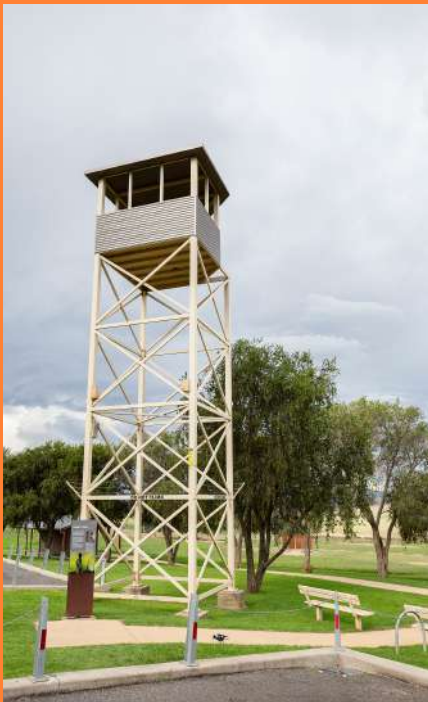
Cowra Camp Replica Guard Tower
